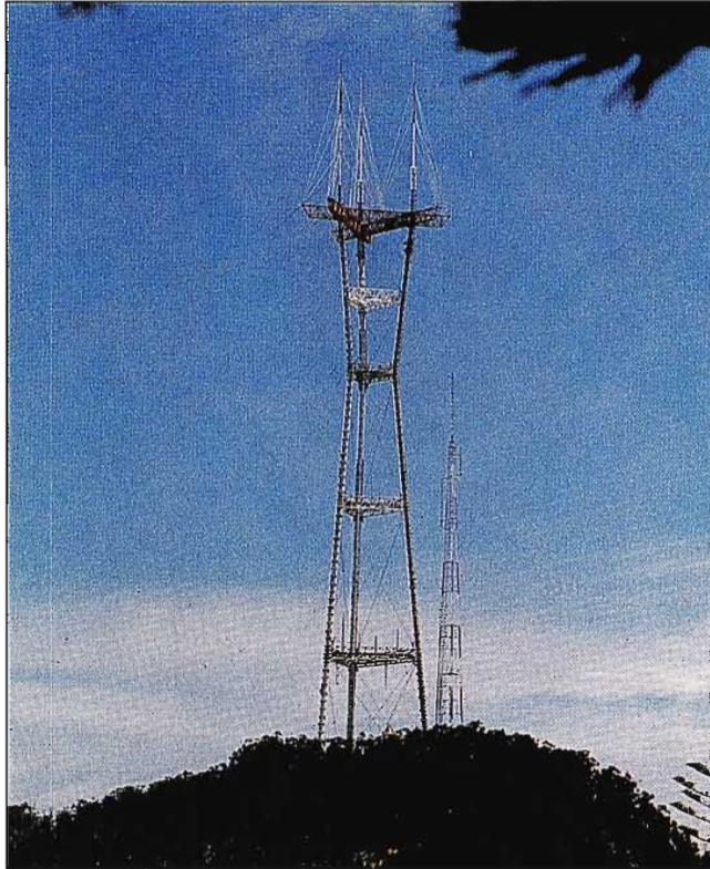
Mt. Sutro Tower Antenna Array covers San Francisco Bay Area.
